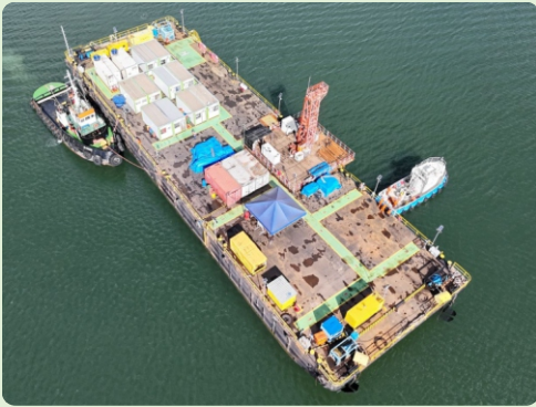
Diagonal Overhead View Operation Site
