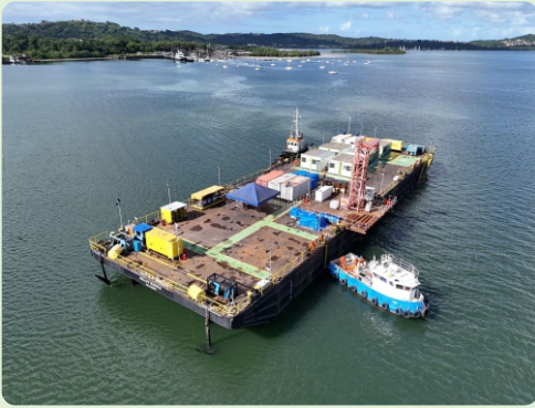
Diagonal Overhead View Operation Site
